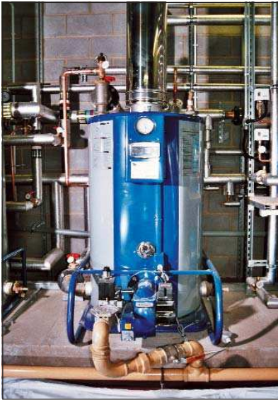
KDB-1035S natural gas installation
