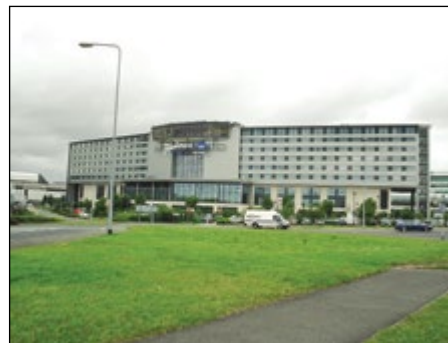
SAS Radisson Hotel, Manchester Airport Expresso
